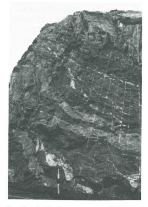
Parallel drillholes after pre-splitting
