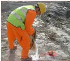
ANFO is the most prevalent explosive used in mining because it is the least expensive and the safest to transport and handle. ANFO type explosives are susceptible to water and, therefore, are not suitable for wet blastholes.
