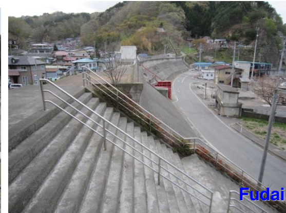
The 15.5m-high seawall was undestroyed in Otobe district, Fudai village, Iwate Pref.
