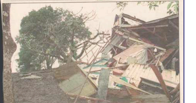
BELOW: A HOUSE is left in ruins in the aftermath of the eruption of a mud volcano in Piparo early yesterday morning. This house was pushed over by the wall of mud on the left.
