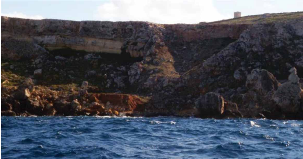
Figure 7. Sinkhole located at Ghadira Bay.
