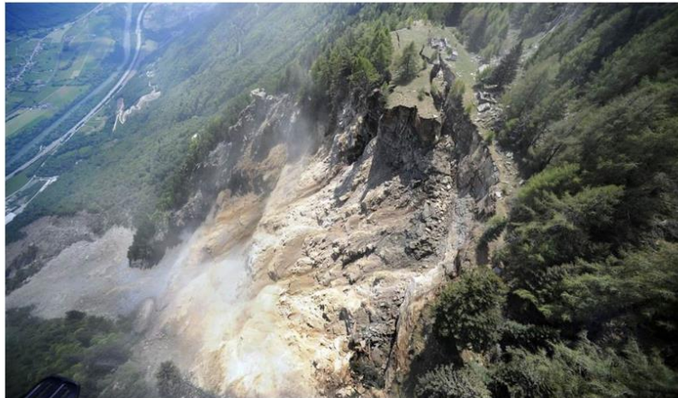
Fig. 10 Rock collapse, Preonzo, Switzerland (Courtesy of S. Löw, ETH, Zurich)
