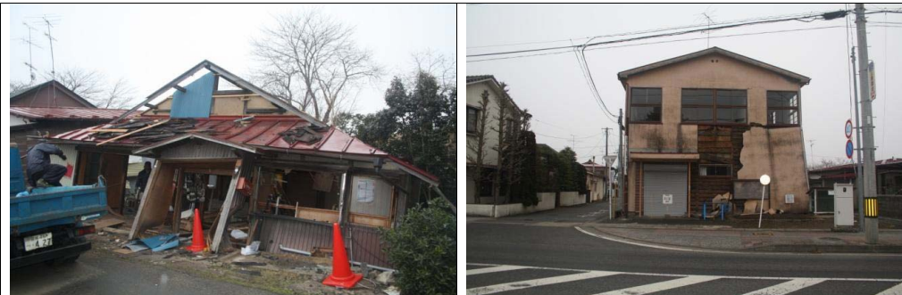
Photo 7: Damage of houses in urban area of Wakayanagi-machi
