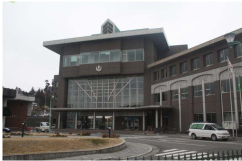
(a) Overall view of the Kurihara City Municipal Office Building
