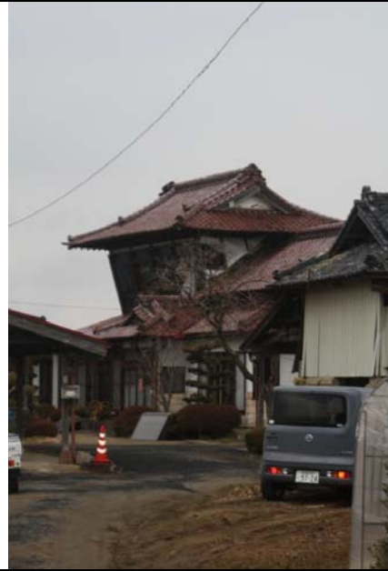
Photo 14: Tiling of the second story of a timber house
