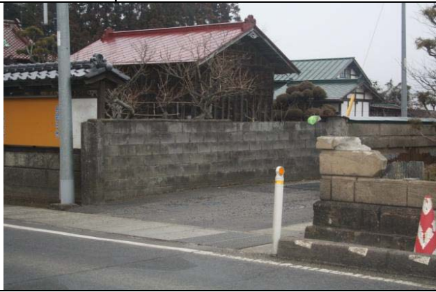
Photo 6: Undamaged concrete block walls and damaged masonry walls
