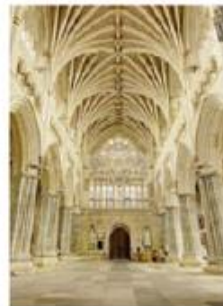
Rib vaulting, Exeter Cathedral, Exeter UK (architect unknown, 1400)
