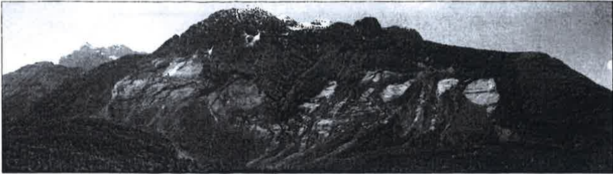
Fig. 4. The failure surface of the 1963 Vaiont Landslide (Mount Toc behind)
