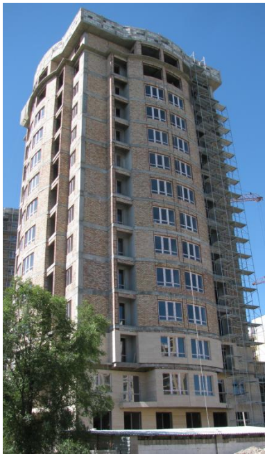
14-floor RC frame with masonry infill
