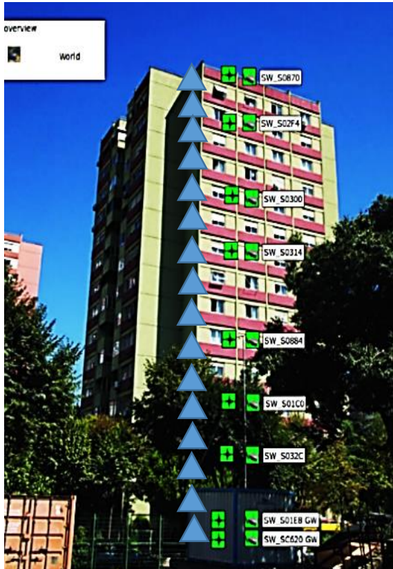
16 story residential tunnel formwork building in Istanbul, Turkey
