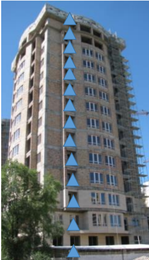
13 storey reinforced concrete building in Bishkek (Kyrgyzstan) Ambient vibration measurements
