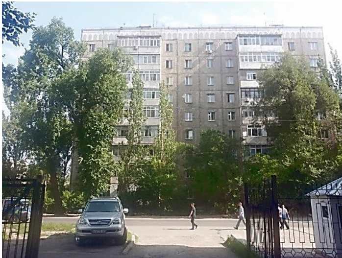
9 storey baseisolated panel building in Bishkek (Kyrgyzstan)
