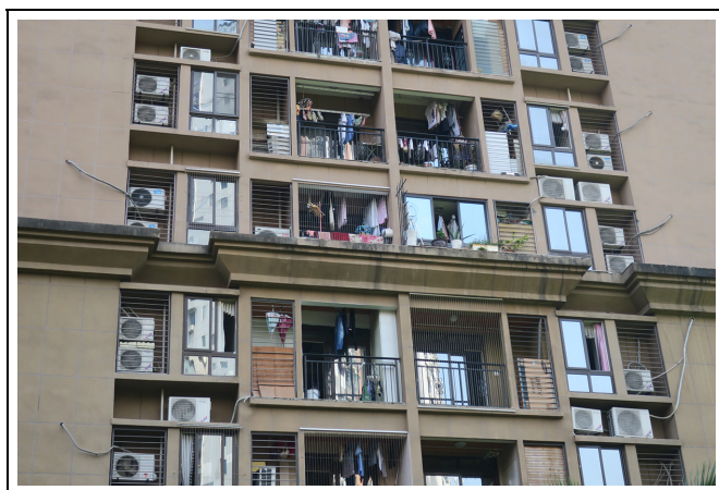
Figure 2. Split units are omnipresent on the facades of high-rise buildings as few new constructions provide central air-conditioning systems.
