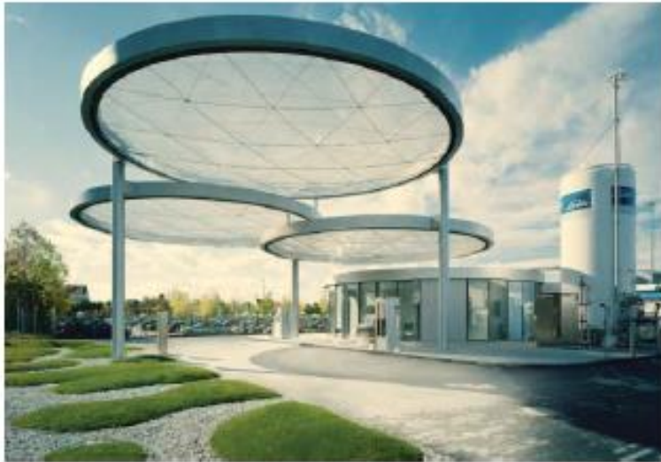
Figure 7.5 Linde hydrogen refuelling station in Munich. (Reprinted by kind permission of Linde AG, Germany.)
