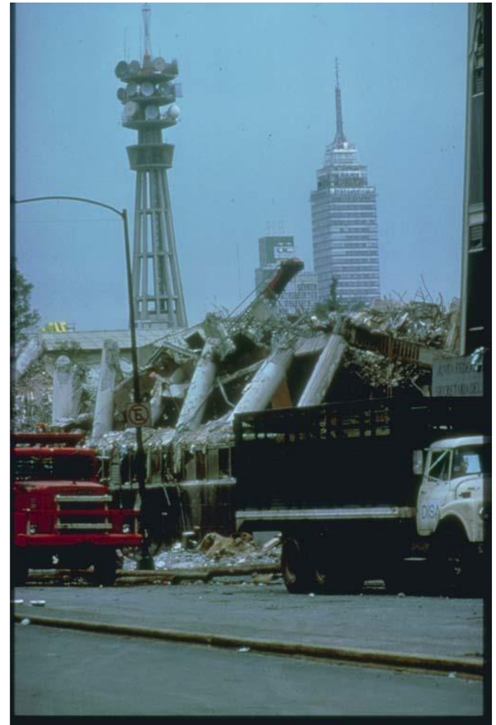
Totally destroyed office building in the foreground, while the 44-floor Torre Latinoamericana office building, in the background on the right, stands
