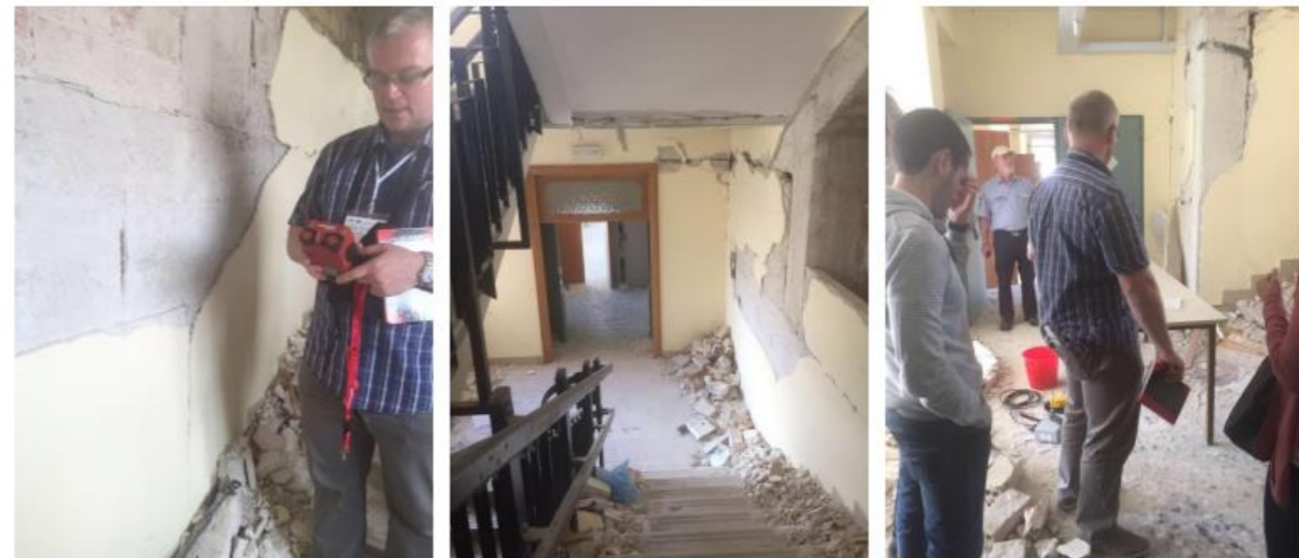
Figure 2: Some images of the building surveyed as part of the demonstration of the methods under development within SIBYL.
