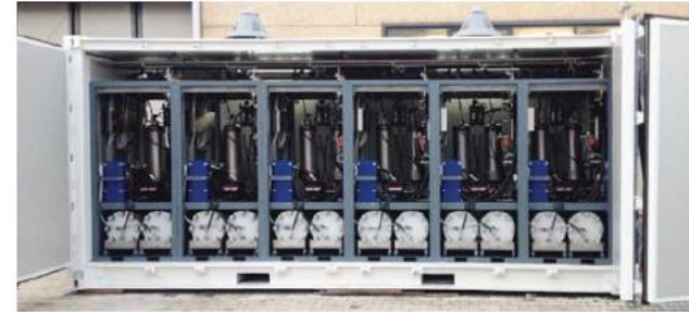
Figure 7.20 McLyzer 60, McPhy aggregates hydrogen production skid units to create larger-output hydrogen production units of 60 \text{ Nm}^3 \text{ h}^{-1} at 12 bar) allowing optimization
