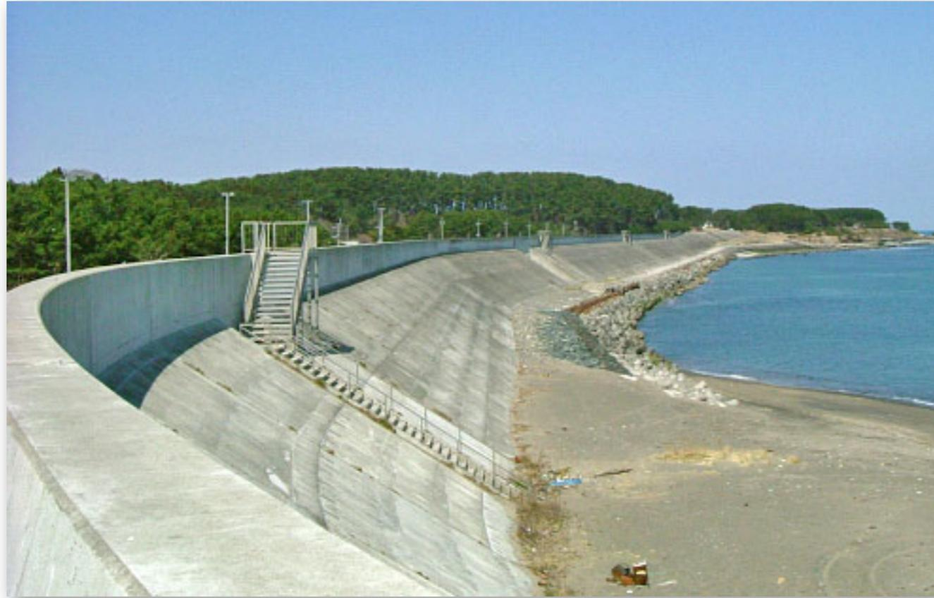
Sea wall with stairway evacuation route used to protect a coastal town against tsunami inundation in Japan.
