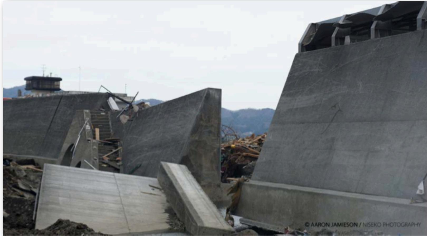
The 2.4 km long tsunami wall in Miyako, Iwate Prefecture, was destroyed. The 6 m, 2 km long, wall in Kamaishi, Iwate Prefecture, was overwhelmed but delayed the tsunami inundation by 5 minutes.
