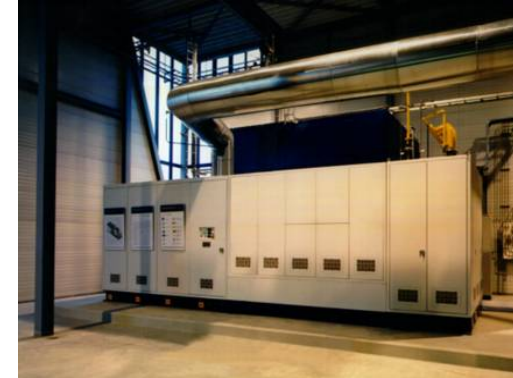
Siemens-Westinghouse 100kW SOFC
