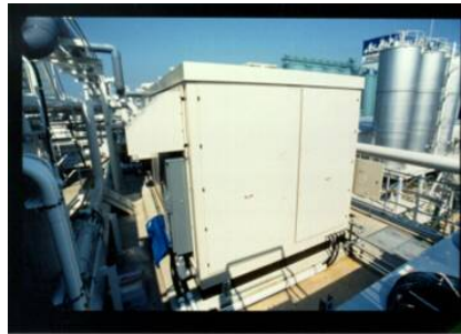
UTC Fuel Cells 200kW PAFC
