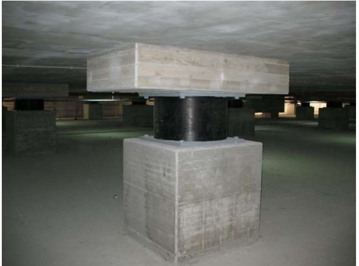
Isolatore in gomma HDRB (High Damping Rubber Bearings)
