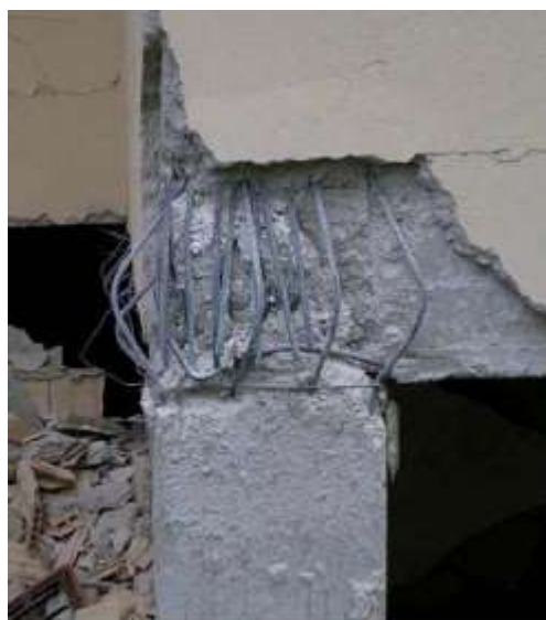
Column sidesway mechanism
