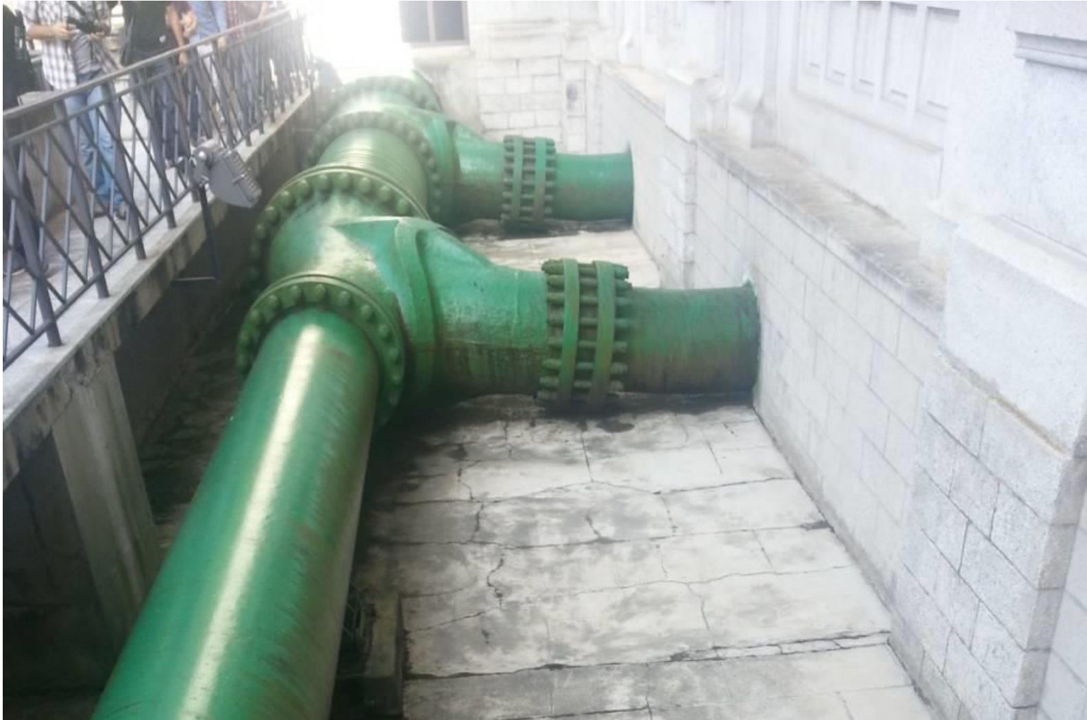
Penstock inlet in the powerhouse
