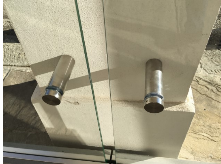
Type A Point fixings with holes
