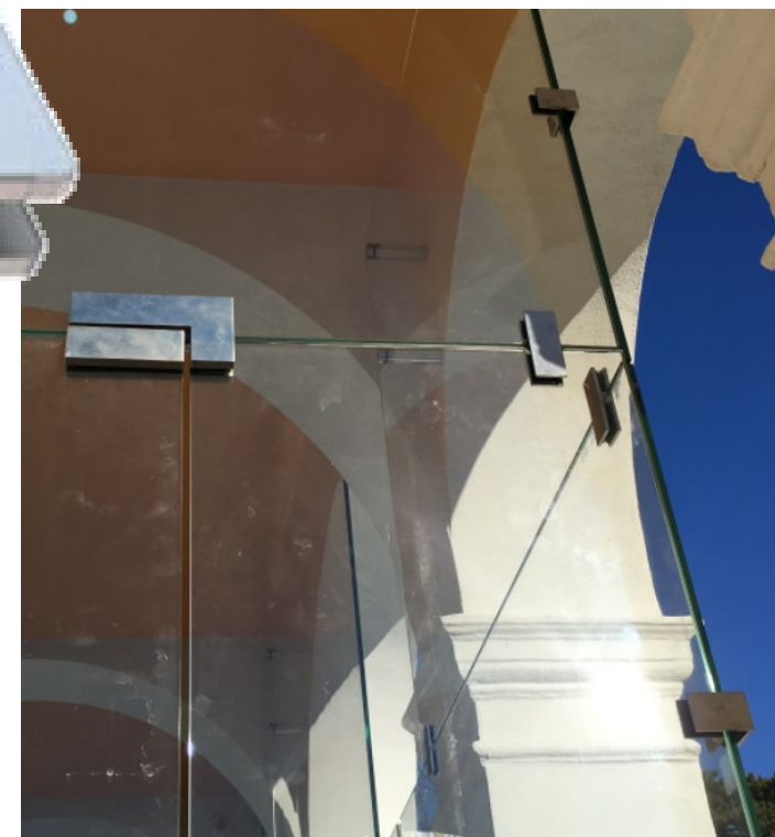
Type C Friction clamps (overlapping plates)
