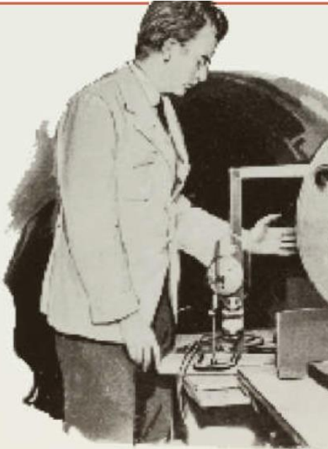
John Logie Baird working on an electromechanical television. In this experiment, he is scanning his hand with the Nipkow disc and broadcasting the image by radio.
