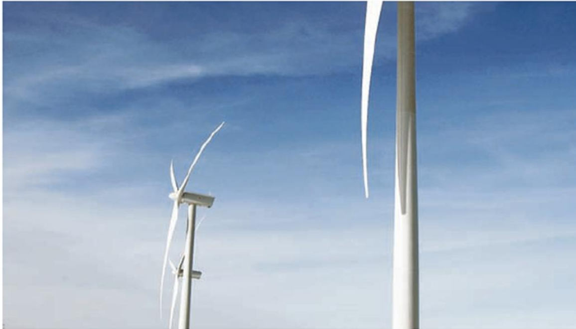
Blades bending close to tower
