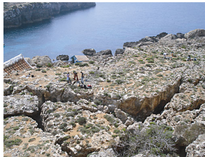
Fig. 5 The rock blocks detached from the limestone plateau, as a result of block sliding, determine a hazard conditions for the tourist infrastructure located beneath
