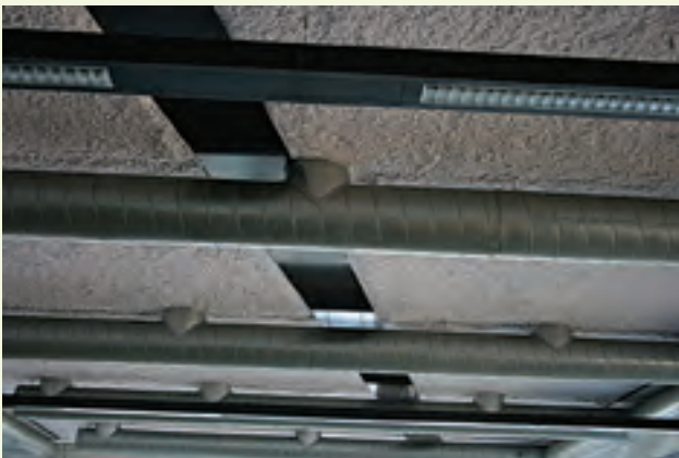
Acoustic fire and thermal treatment. PHOTO: D HES
