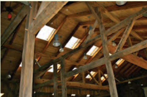
Demolished old barn becoming a library.
