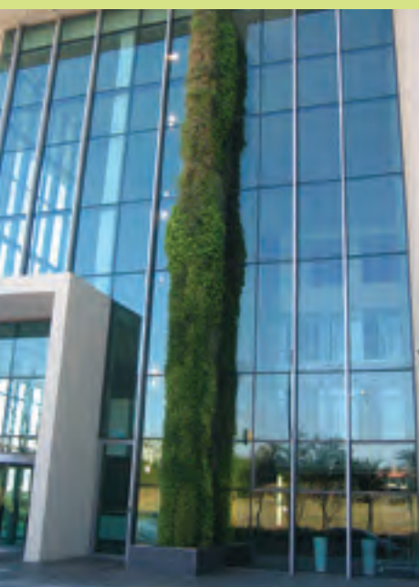
Figure 5: The ultimate in green bling – Africa's highest green wall (to date), Nedbank Falcon Building. PHOTOS: C DU PLESSIS
