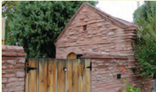
Old stone maintenance building.
