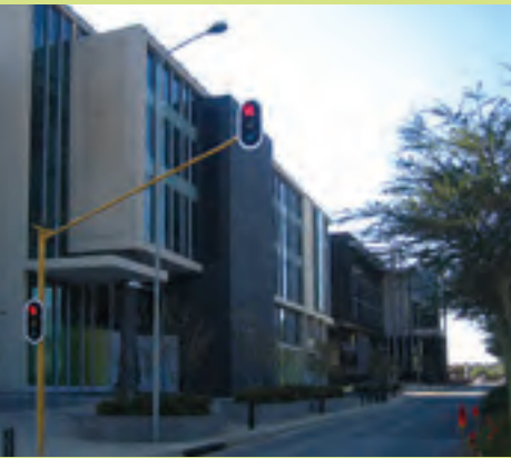
Figure 3: Nedbank Falcon Building (Architects: Boogertman and Partners)
