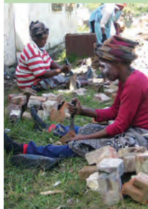
Women cleaning bricks for re-use PHOTO: V COLLIS
