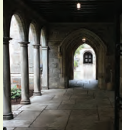
Colonnades, secure protected path, connection of spaces PHOTO: D HES
