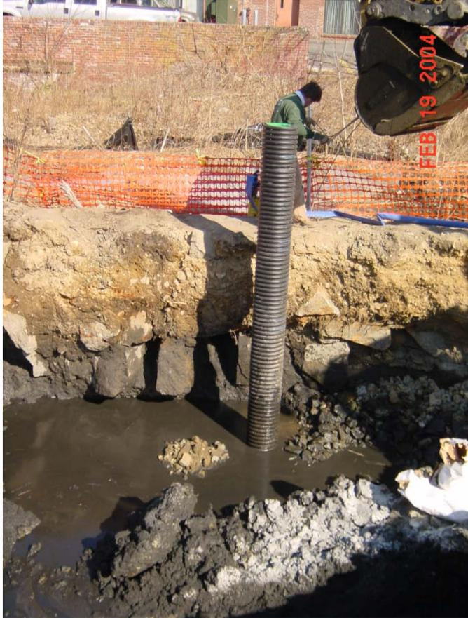
Small, side pit dug into corner of large pit for sludge/polymer mixing.
